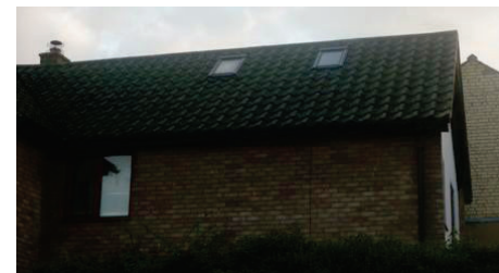
Existing rooflights at 68 Maids Causeway
