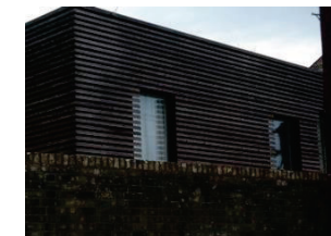
Stained Weatherboards at 16 Auckland Road
