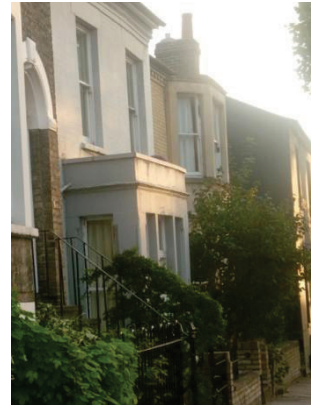
Flat roof projection at 54 Maids Causeway
