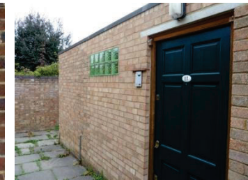
Glass blocks in nearby rd
