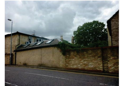
Even higher wall adjacent buildings on West side of Fitzroy Street
