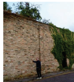
High wall in adjacent street
